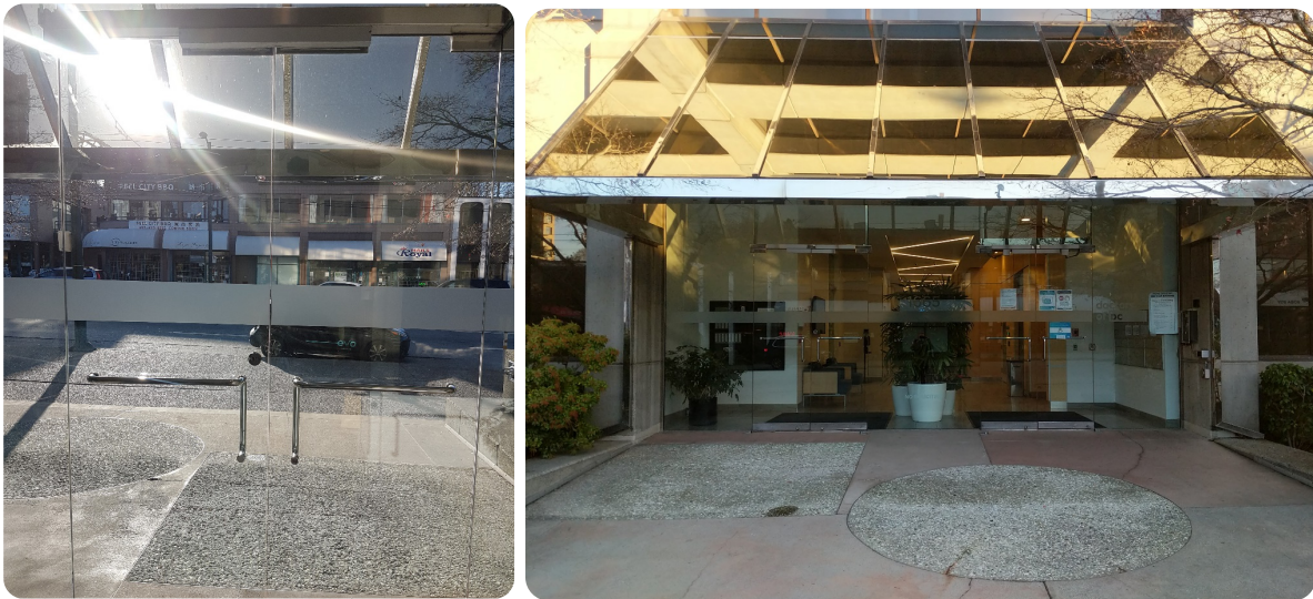
Figure 3.1-3: Lobby doors (left) and lobby viewed from building exterior (right)
