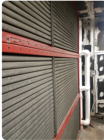
Figure 3.3.1-3: AHU1 heating coil
