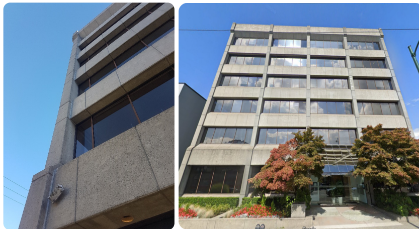
Figure 3.1-1: Exterior: main façade (left) and building front view (right)
