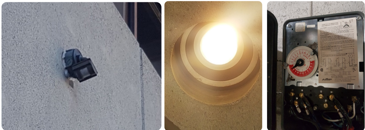
Figure 3.2-12: Exterior lighting: photocell (left), canopy potlight (centre), and timer (right)
