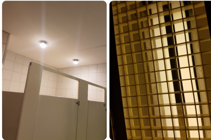
Figure 3.2-4: Typical women’s washroom lighting: 2-lamp 2-pin CFL pot light (left) and 2-lamp 4-pin LED Sconce (right)
